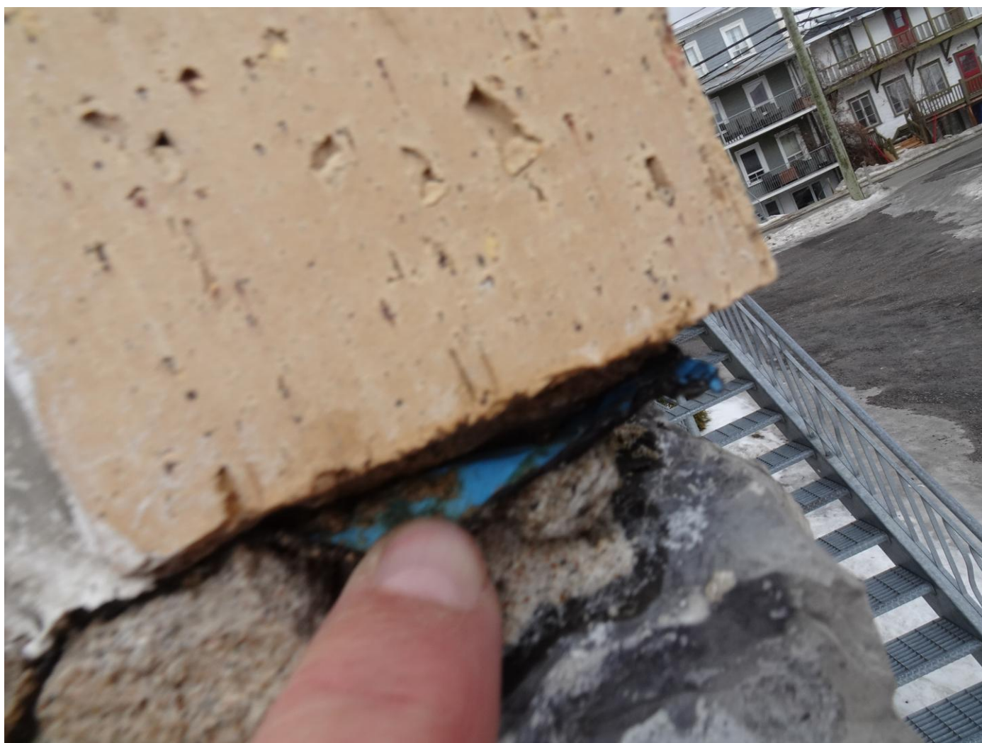
Photo 6: membrane bitumée (blues keen).
